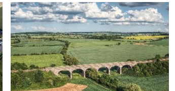
Railways/Steam Trains – Ackworth Six arches railway bridge.
